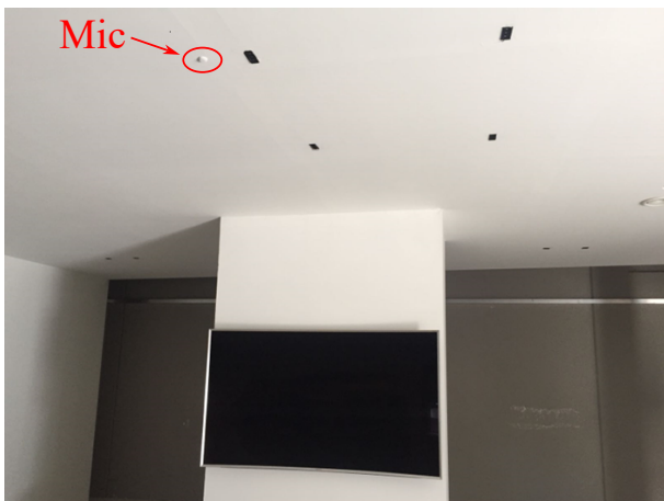
Figure 8: Installation of the microphone in the roof near the listener position.
