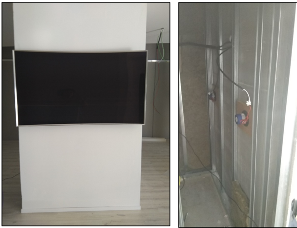
Figure 7: Installation of the vibrating sound transducers behind the wall where the TV is installed.
